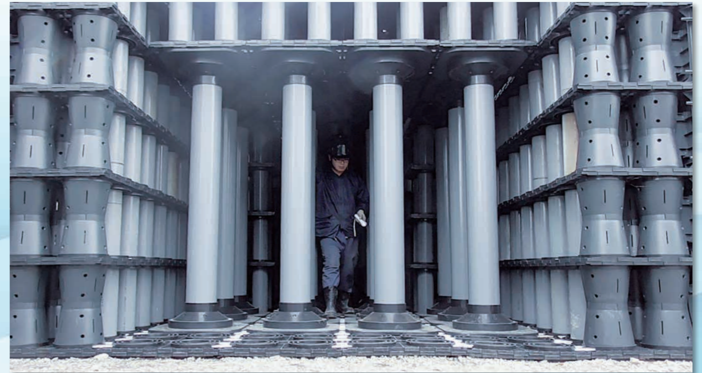
▲ Aqua Palace assembled to have a capacity of about 100m 3 .
