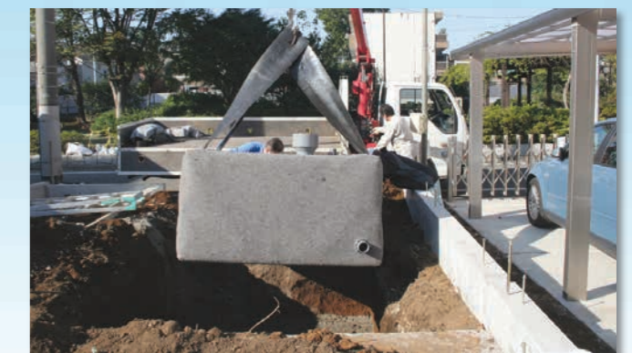
▲ Small parts are assembled in the plant, transferred to the construction site and lifted by a crane.
