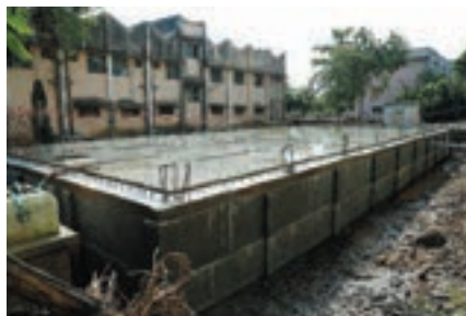
5 Completion of concrete placement
