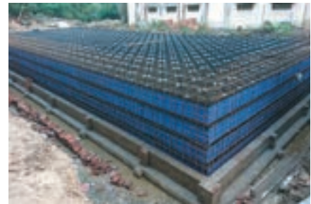
3 Install inner form plastic cardboards
