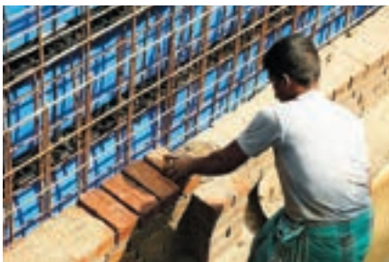
4 Bricks (outer formwork) pile construction
