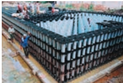
2 The SP main pipes are erected in the central part.
